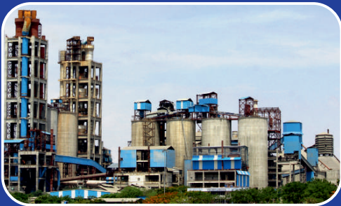
CEMENT PLANT MUKTYALA
