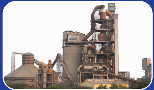
CEMENT PLANT MACHERLA
