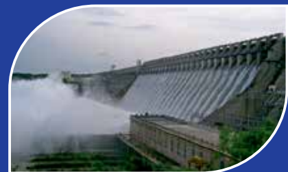
NAGARJUNA SAGAR DAM
