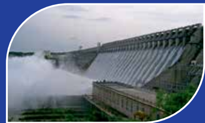
NAGARJUNA SAGAR DAM
