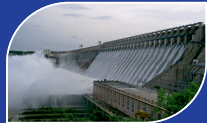
NAGARJUNA SAGAR DAM
