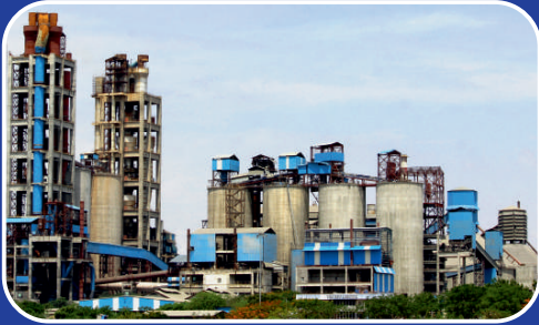
CEMENT PLANT MUKTYALA
