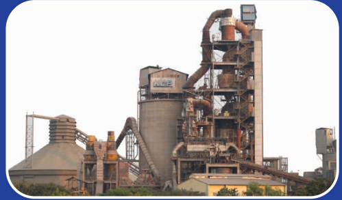
CEMENT PLANT MACHERLA
