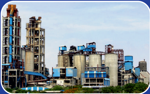
CEMENT PLANT MUKTYALA
