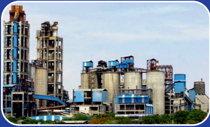
CEMENT PLANT MUKTYALA
