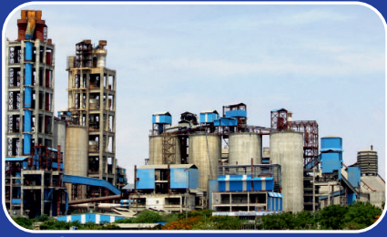
CEMENT PLANT MUKTYALA
