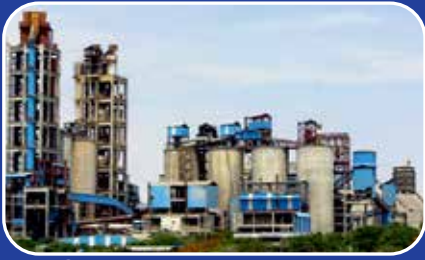
CEMENT PLANT MUKTYALA
