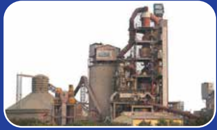
CEMENT PLANT MACHERLA
