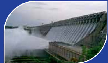
NAGARJUNA SAGAR DAM
