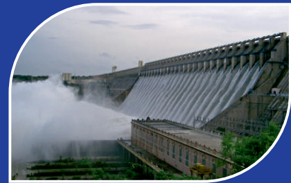
NAGARJUNA SAGAR DAM
