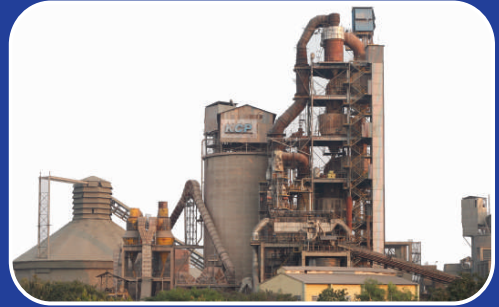
CEMENT PLANT MACHERLA
