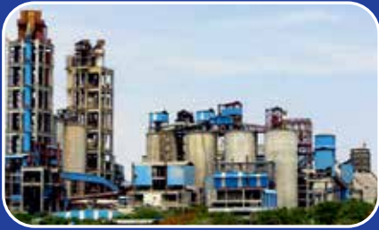
CEMENT PLANT MUKTYALA
