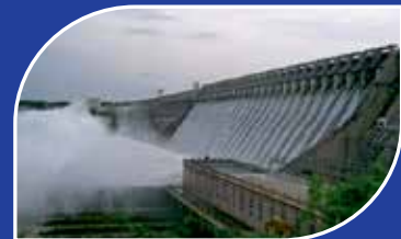
NAGARJUNA SAGAR DAM
