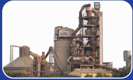
CEMENT PLANT MACHERLA
