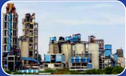
CEMENT PLANT MUKTYALA
