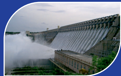
NAGARJUNA SAGAR DAM
