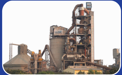
CEMENT PLANT MACHERLA
