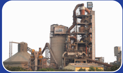
CEMENT PLANT MACHERLA
