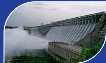
NAGARJUNA SAGAR DAM
