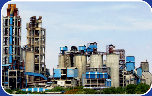
CEMENT PLANT MUKTYALA
