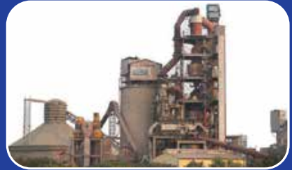
CEMENT PLANT MACHERLA
