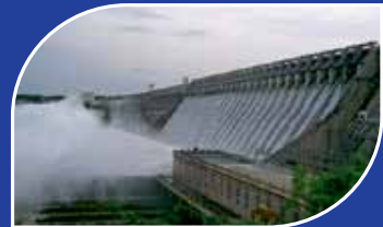
NAGARJUNA SAGAR DAM
