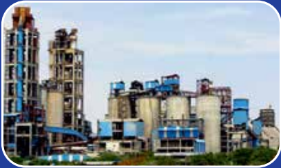
CEMENT PLANT MUKTYALA
