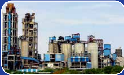
CEMENT PLANT MUKTYALA
