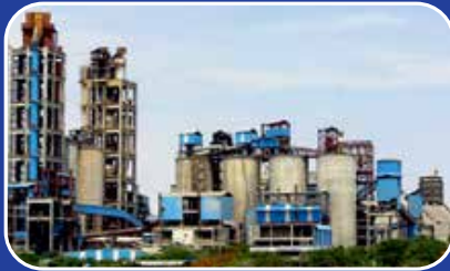
CEMENT PLANT MUKTYALA
