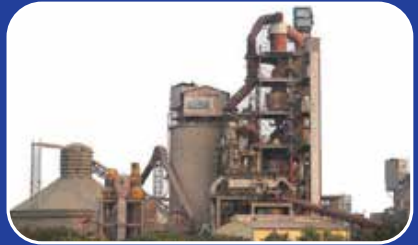
CEMENT PLANT MACHERLA
