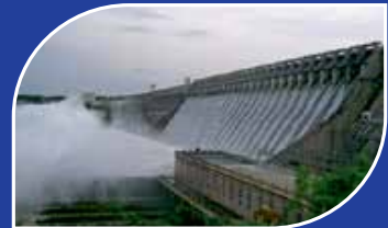
NAGARJUNA SAGAR DAM
