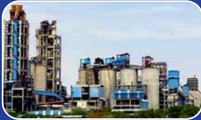
CEMENT PLANT MUKTYALA
