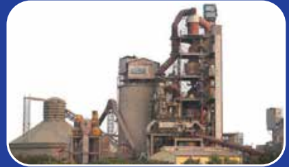
CEMENT PLANT MACHERLA
