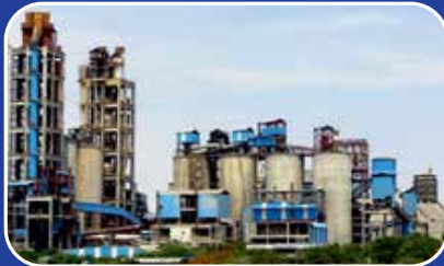
CEMENT PLANT MUKTYALA
