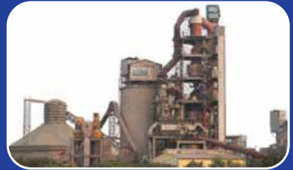
CEMENT PLANT MACHERLA
