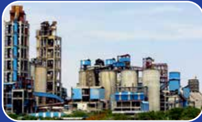
CEMENT PLANT MUKTYALA
