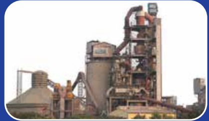
CEMENT PLANT MACHERLA
