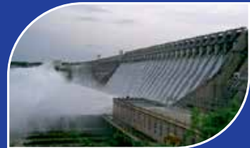
NAGARJUNA SAGAR DAM
