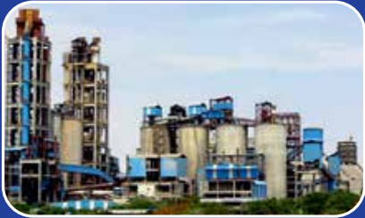
CEMENT PLANT MUKTYALA
